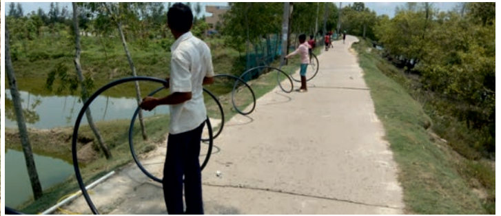
Laying 1300 mtrs. long underground water line from our old school premises at Parasmani to RVPS School at Santigachi, Sundarbans
